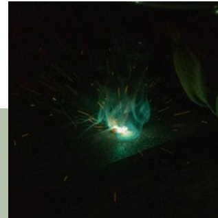
Re-weld the grinded zone
