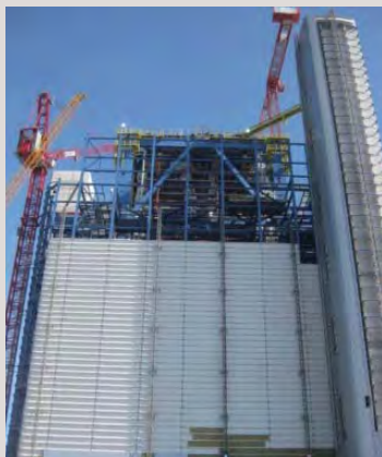
E-on power station, near Rotterdam, The Netherland
