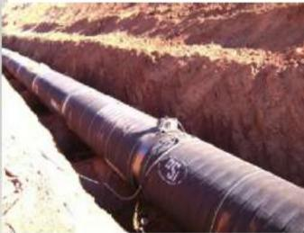
Gullco PIPE KAT® Automated Pipe Welding System with integrated wire feeder
